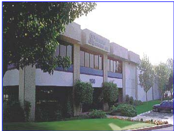
In a 65,000 square foot facility, SC Hydraulic is capable of setting the industry's highest standard while maintaining the best delivery times
